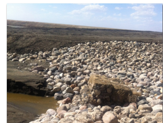
More rock added at an erosion control drop structure.
