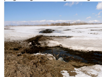
Culverts cleaned out early spring.
