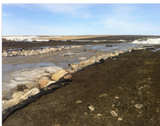
More geo-tech fabric and rock needed to be added to the sides of the ditch.
